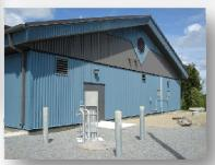
KAL provided engineering services to design the Kingfisher Lake Water Treatment Plant. The facility utilizes a dual train conventional water treatment system with full redundancy. The maximum design flow for each water treatment train is 4.65 litres/sec (402 m³/day). Each treatment train produces safe drinking water meeting O.Reg 170/03 at all possible flow rates equal to and less than 4.65 litres/sec.
