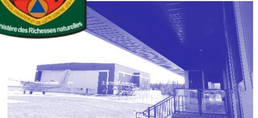
KAL provided design and contract administration services for a new, two storey office building added on to the existing MNR Dryden Fire Management Centre (FMC). The combined floor area of the new office space is 14, 478 ft<sup>2</sup>. In order to connect the new works to the existing FMC alteration and renovation work was required to the FMC.
